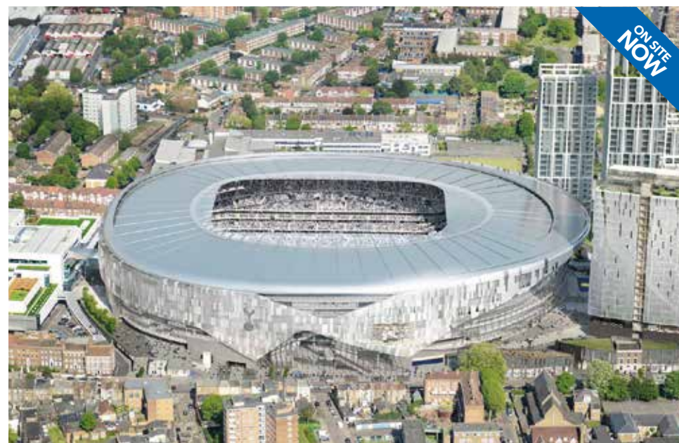
6 Circa £750m Tottenham Hotspur stadium development
