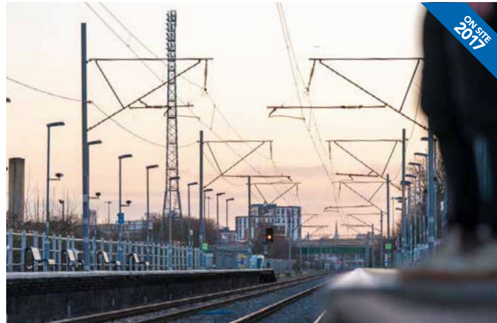
3 £121m West Anglia Main Line upgrade to increase train frequency connecting Tottenham to Stratford
