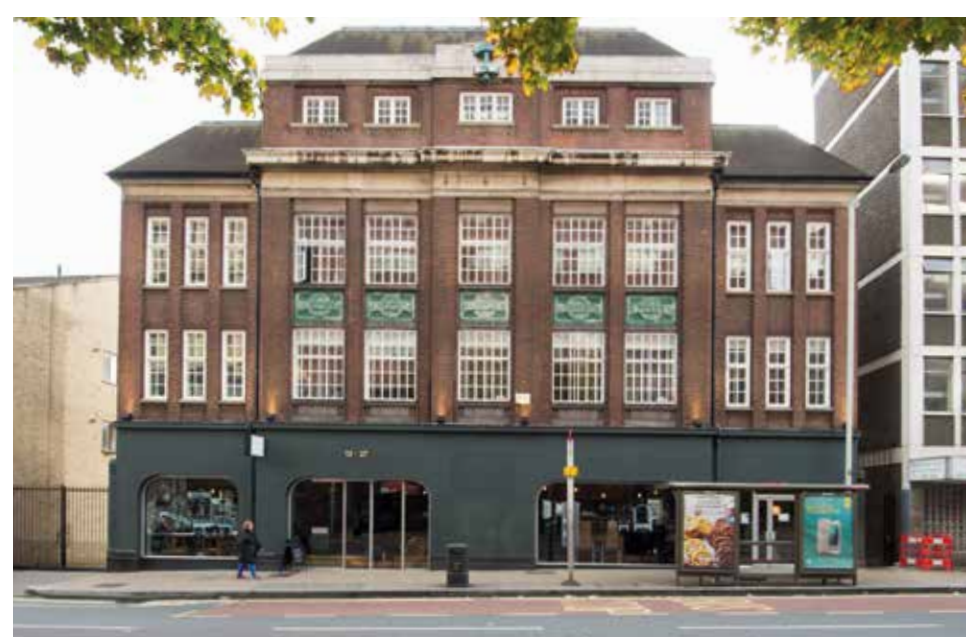
2 Green Rooms - the UK's firsts arts hotel, a social enterprise offering affordable accommodation housed in an art deco building
